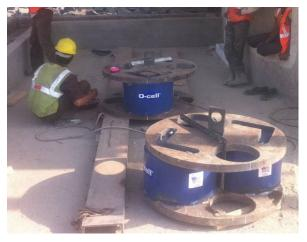
O-cell Assembly Fabrication
